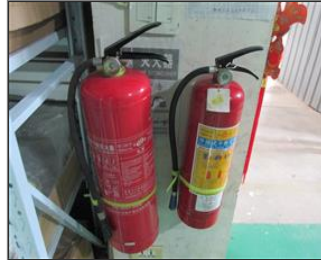
Photo of fire safety equipment Fire extinguisher.JPG
