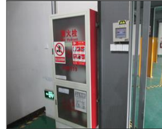
Photo of fire safety equipment Fire hydrant.JPG
