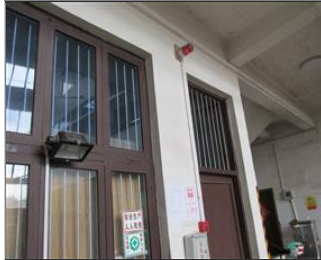
Photo of fire safety equipment Fire alarm.JPG
